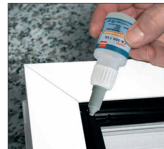
APTK/EPDM seals in window construction
