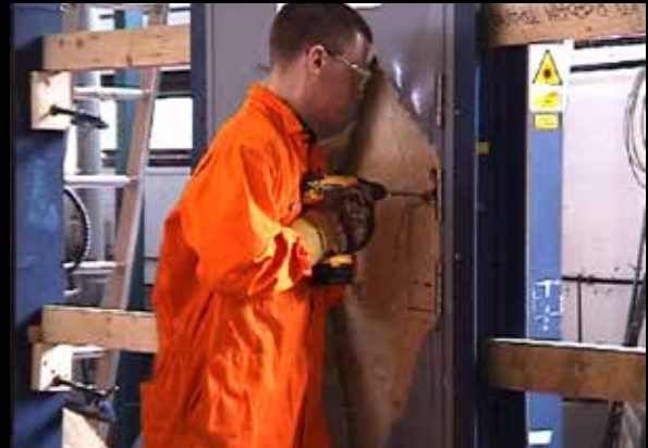
With the door skin removed, a drill is used to attack the hardware.
