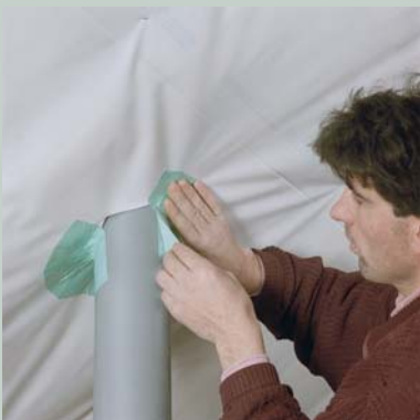
Sealing of penetrations through a vapor barrier with Gerband 586
